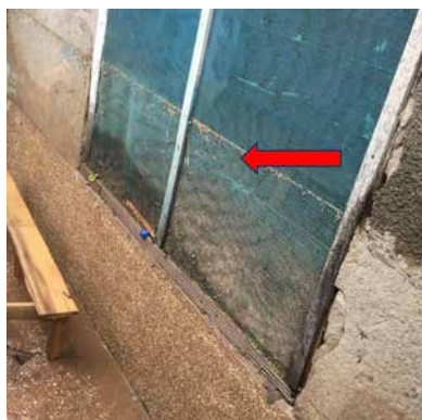
Fig 1. Level of flood water marked on the walls of houses
