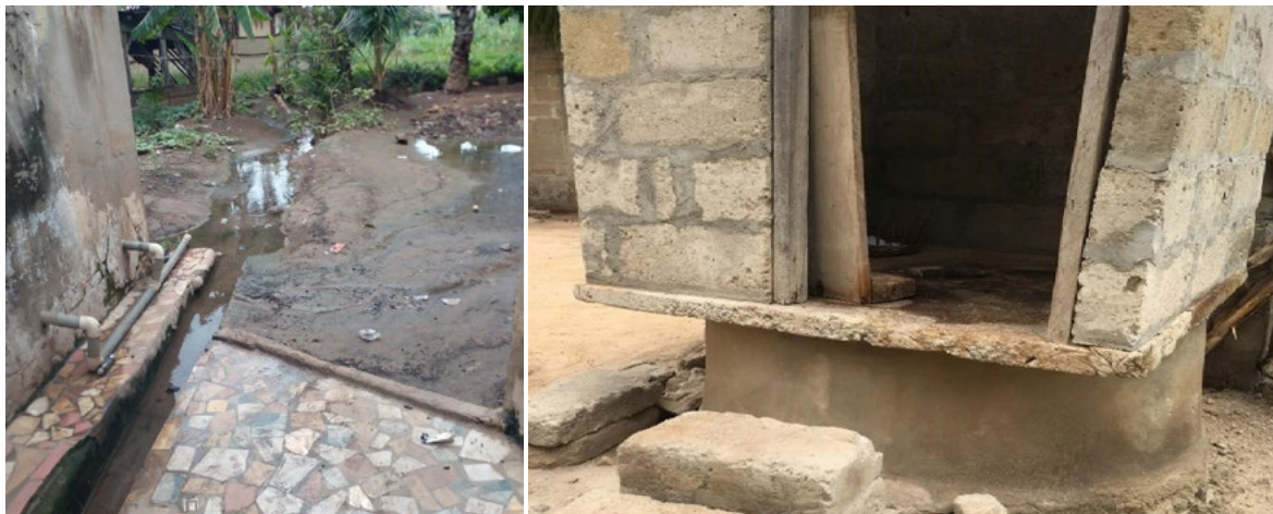
Plate 11: Adaptions Being made as Coping Strategy - Raised Toilet in a House
