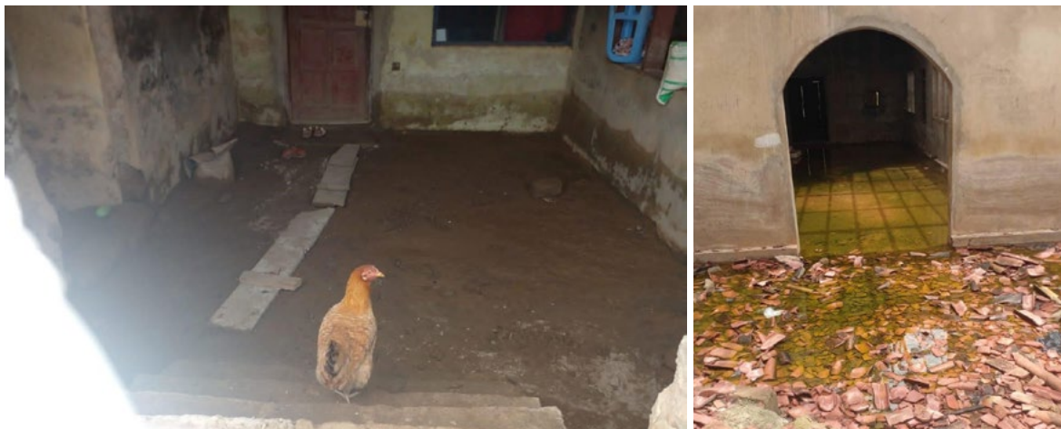
Plate 10: Abandoned Houses After Flood
