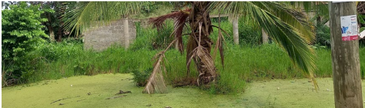
Plate 9: Uncompleted abandoned house at Deduako in Stagnant Flood Water, near KNUST
