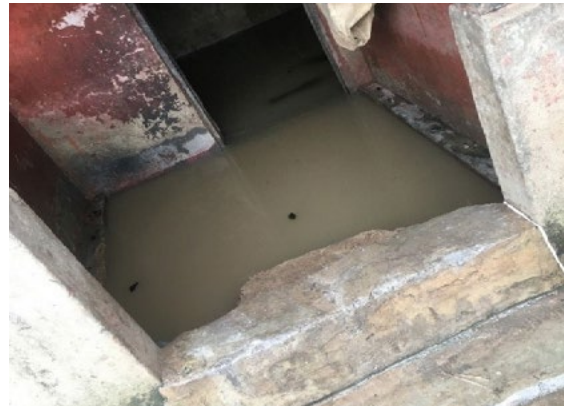
Plate 4: An Elevated Entrance
