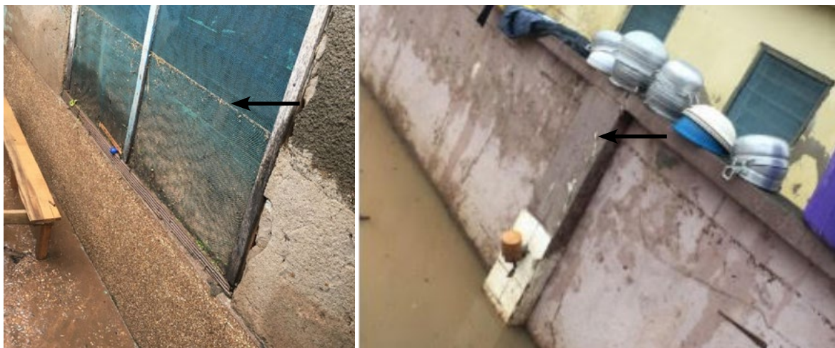
Plate 3 (B): Level of Flood Water Marked on the Walls of Houses
